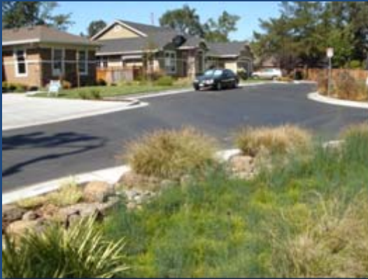
Bio-retention, rain gardens and bio-swales
