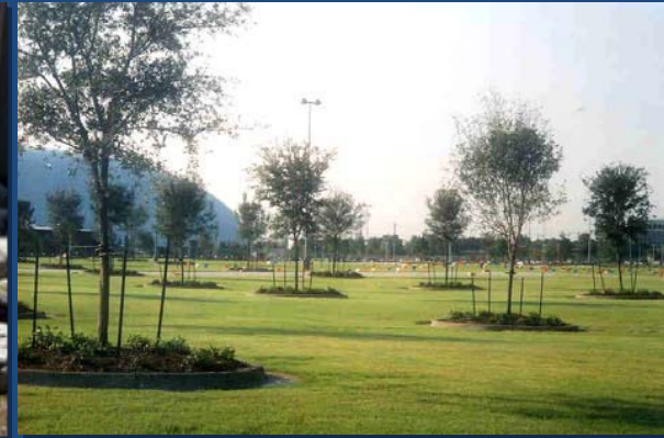
Pervious paving on parking lot
