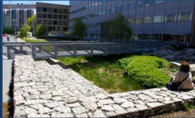
Constructed wetlands within urban development
