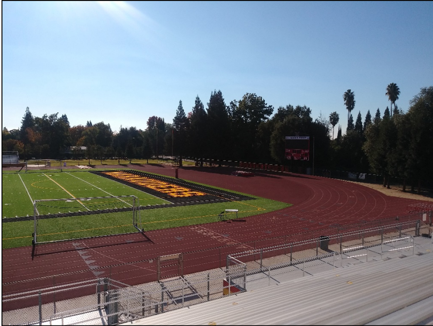
North side of stadium, looking southwest
