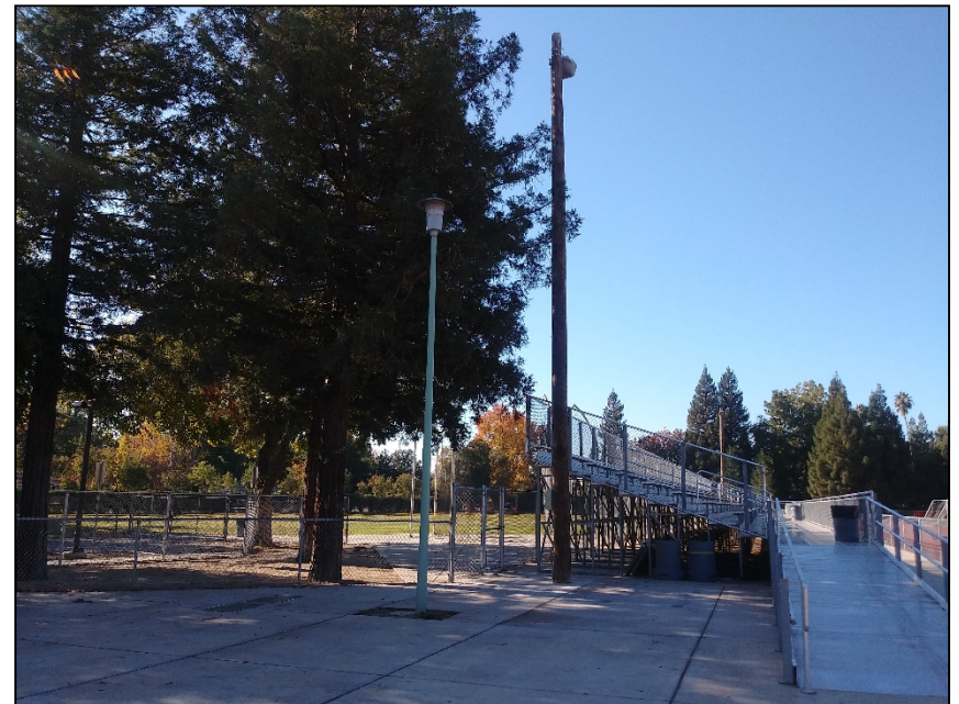
South side of stadium, looking west
