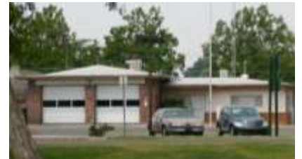
Rio Linda Fire Station showing original brickwork
