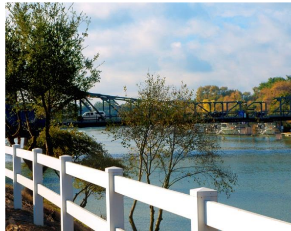
Walnut Grove Bridge Crossing Sacramento River
