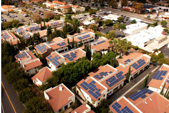
Neighborhood layouts and parcel orientation will encourage solar installations.
