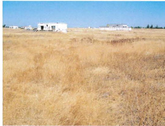
Overview of Structures
